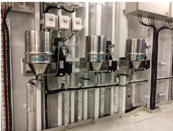
*Three GreenOil filters are installed for each of the three Aux. Engines, which are into the operation instead of the purifiers.*
