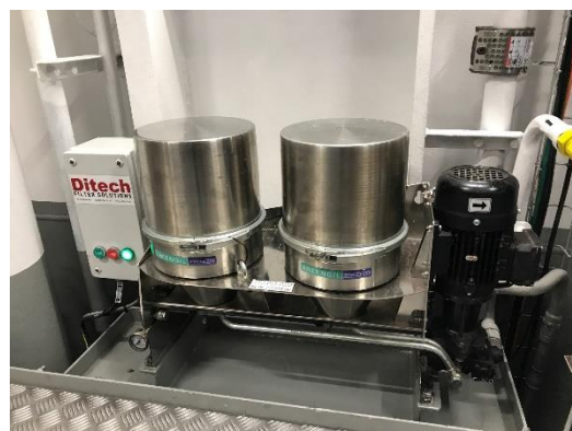
Picture 3. WP1-P2-400 for engine lubrication oil. Photo: Johannes Solsvik
