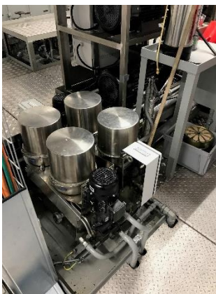
Picture 2. 2x WP1-C1-1000 for diesel filtration and water separation. Photo: Johannes Solsvik
