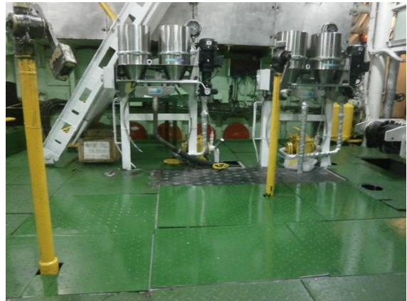
The two GreenOil systems WP1-B2-400 replacing fully the existing purifiers.
