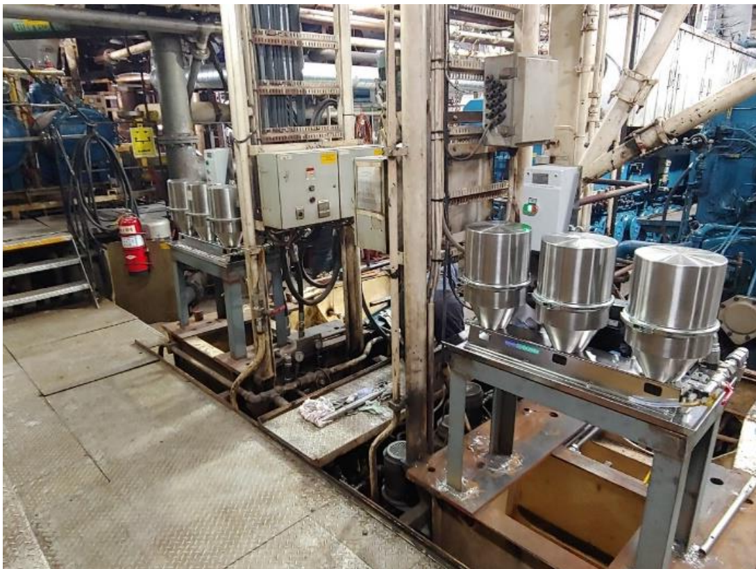
Picture 2. Northern Eagle with the 2x GreenOil WP1-P2-750 for the Bergen BRM 8 main engines. Photo: Troy Bills.
